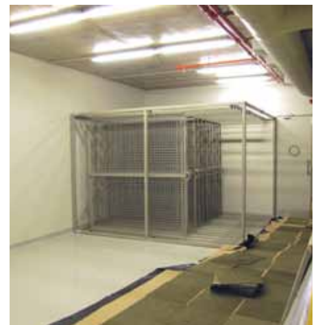
Construction continues at our customised archive facilities
