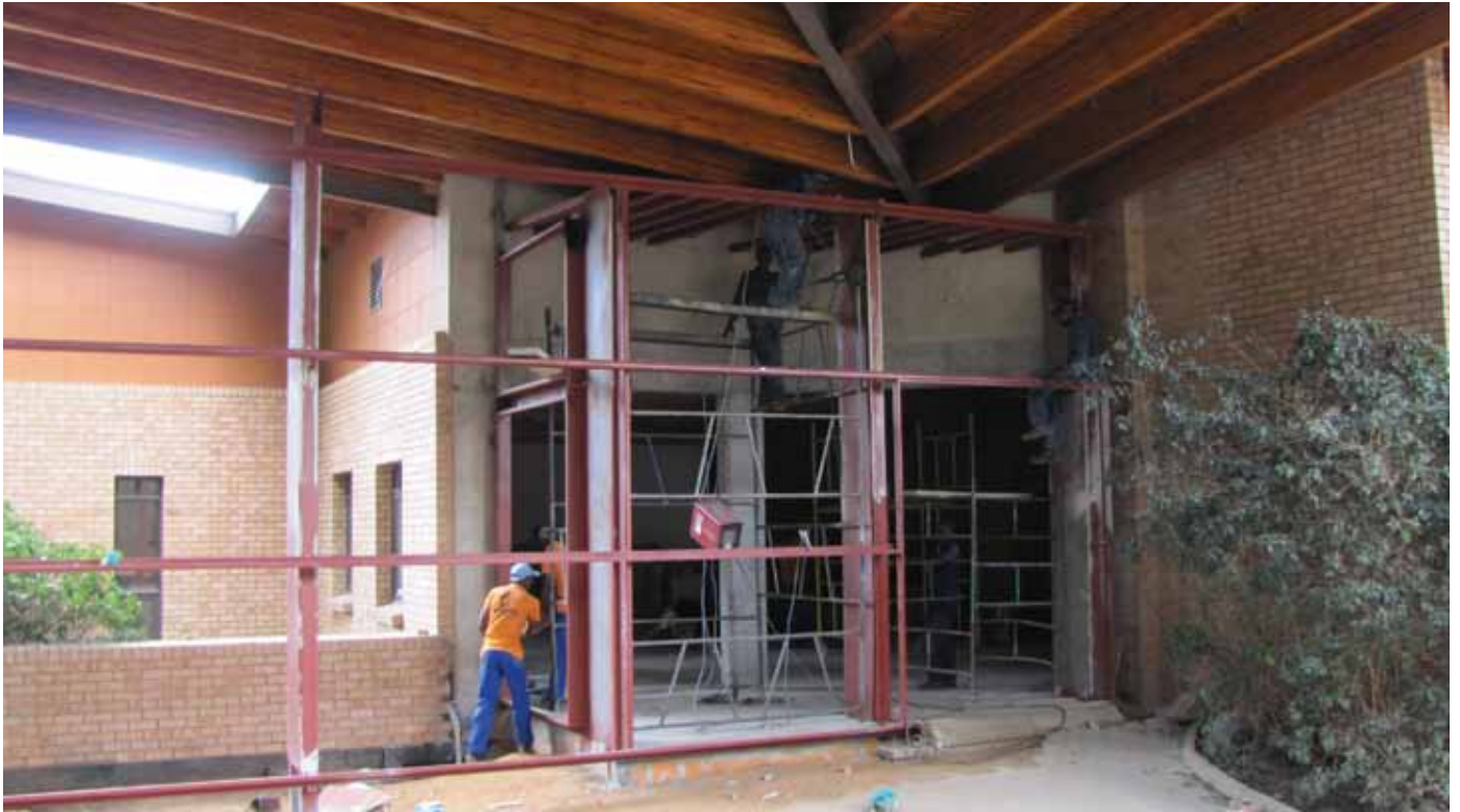
Refurbishment continues at the Foundation premises in Houghton, Johannesburg
